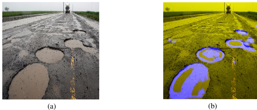
Figure 6. Results from the trained model: (a) original image and (b) predicted segmentation mask
